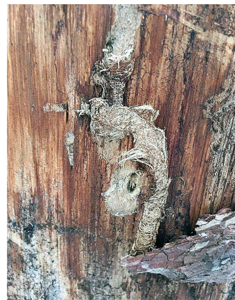
Figure 5. Typical signs of colonisation by xylophagous insects
